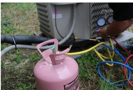
Connect the manifold refrigerant hose to the refrigerant supply tank. Verify the high & low side valves on the manifold are closed before proceeding. Purge the air from the low side.
