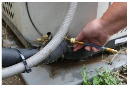
Turn the a/c system on, and verify the unit is running. Connect Dye Inject to the low-side service port of the system (This is generally the large line).
